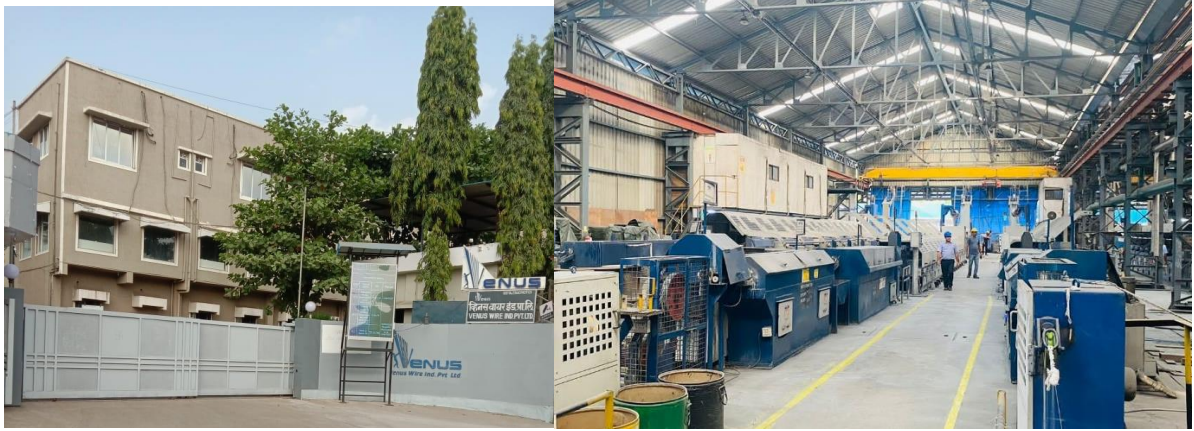
Figure 1 Manufacturing facility of Venus Wire Industries Pvt. Ltd. at Raigad, Maharashtra
